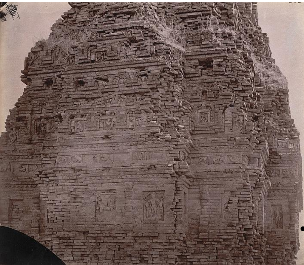
● Close view of bhitargaon temple façade showing the detail of mouldings and sculpture niches.
