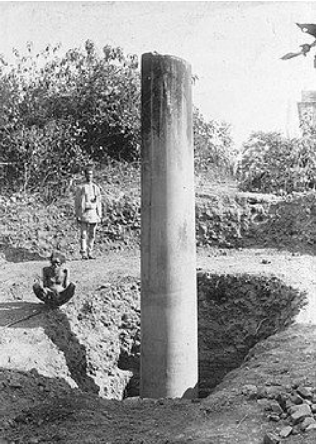
Lumbini pillar, Capital is lost. Horse is believed to have been there.
