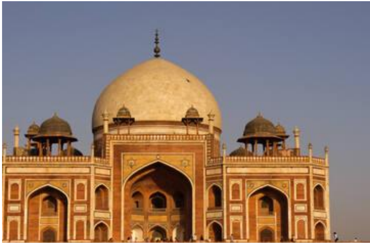
Left- Fully mature form of the double dome is seen, for the first time in India in the tomb of Humayun
