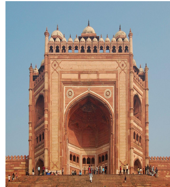
Buland Darwaza at Fatehpur Sikri has a four-centred archway with vaulted iwan.
